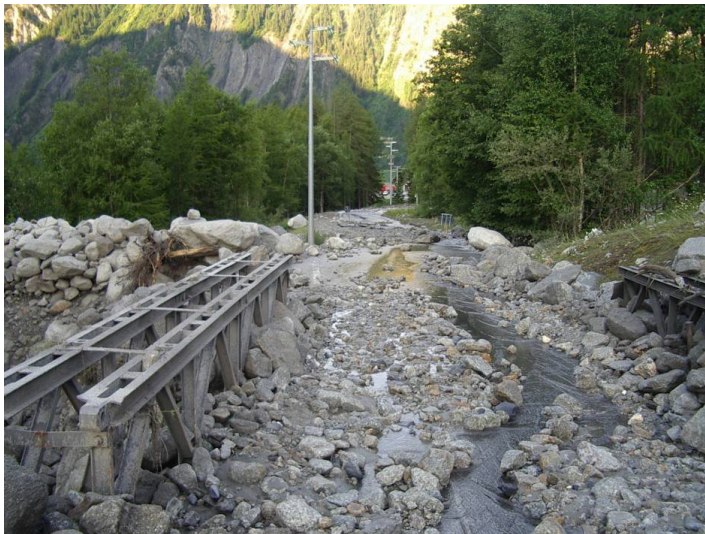
Figure 51: Example of deposition of debris on a regional road caused by the outburst of a water pocket of Rochefort glacier
