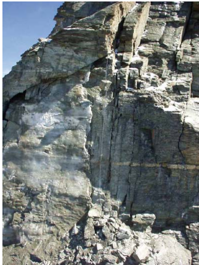
Rockfall scar with exposed ice. Photo: L. Trucco
