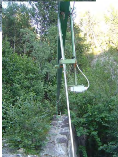
Debris flow alert system
