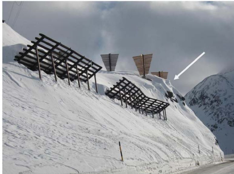
Figure 30 : Kolktafeln, to reduce the formation of cornices above the Berninapass Road in Switzerland. Photo. Gian Cla Feuerstein, AfW Zuoz, Switzerland, 2008
