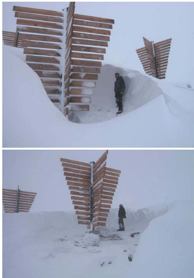
Figure 29 : Kolktafeln prevent the formation of a continuous snow cover, Dimension of the Kolktafel: height = 4 m, largest width = 4 m. Photo. Gian Cla Feuerstein, AfW Zuoz, Switzerland, 2008
