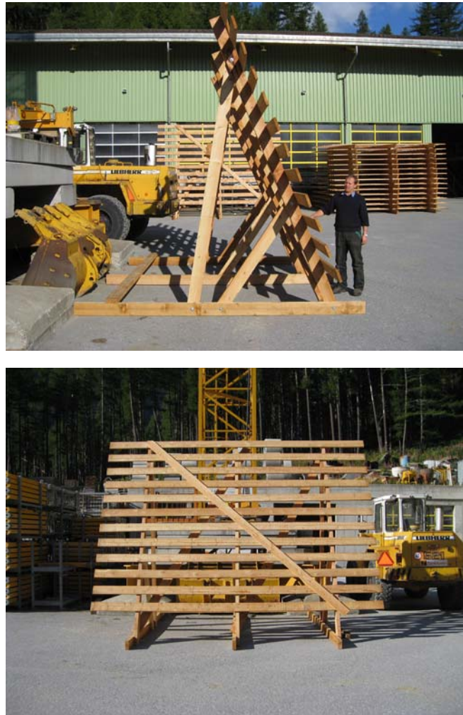
Figure 22 : Snow drift fence with a bottom gap, Type Wyoming, Photo A. Burkard, 2009
