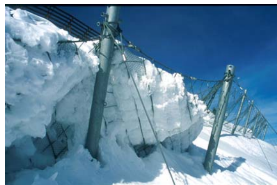
Figure 12 : Snow net type GEOBRUGG
